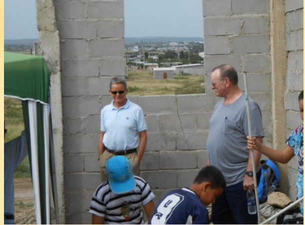
Neighborhood church in Salinas being built.
